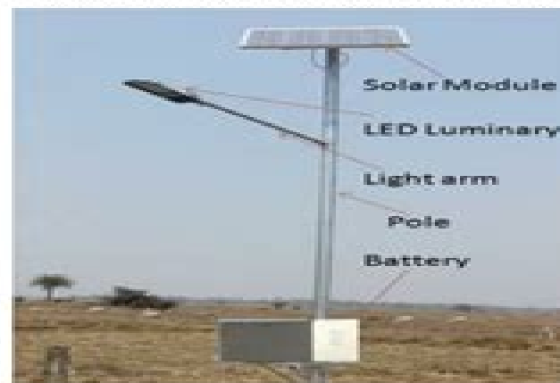
Figure 1 Stand alone Solar streetlight
